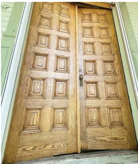
▲ Along with the overall project, doors and windows demanded a lot of attention to detail.
