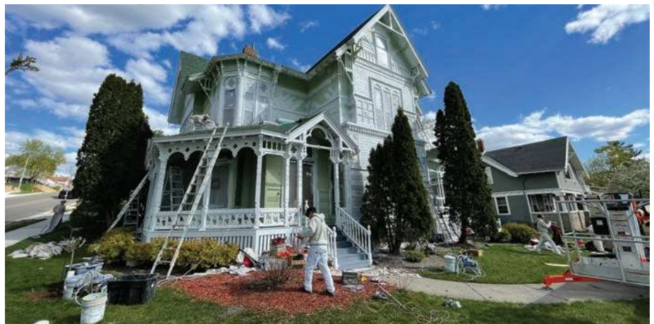
▲ Safety was paramount in reaching the upper floors.
