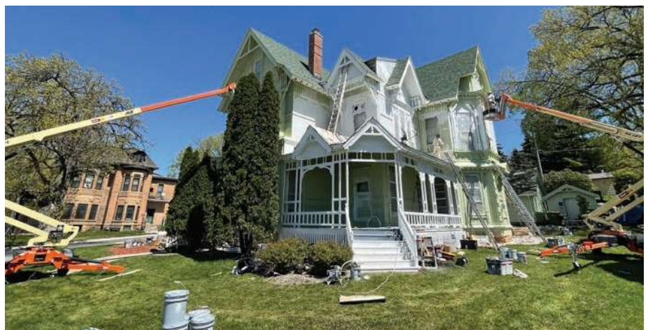
▲ Lifts brought the crew to the upper floors.
